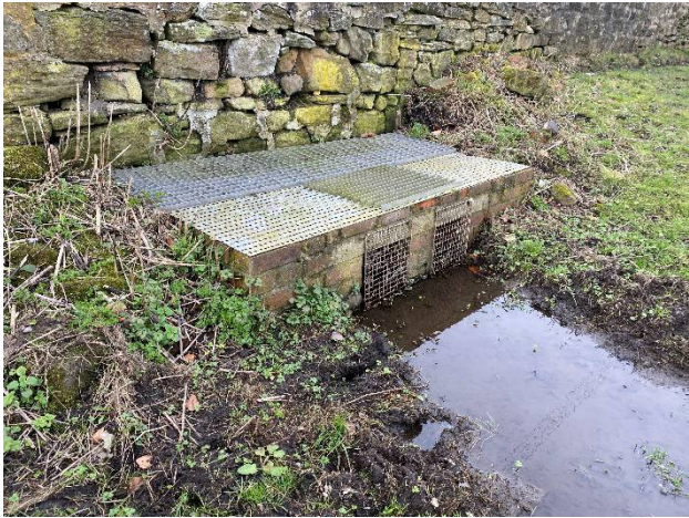
Photo 1: Culvert under Lamesley Road (TN2)
